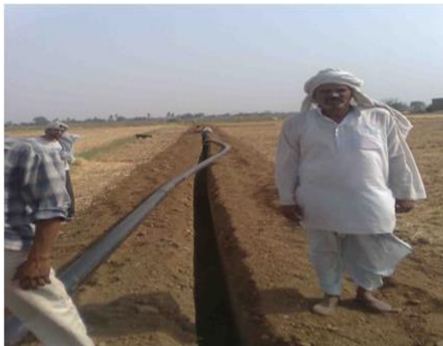
Under Ground Pipe Line being laid in Haryana
