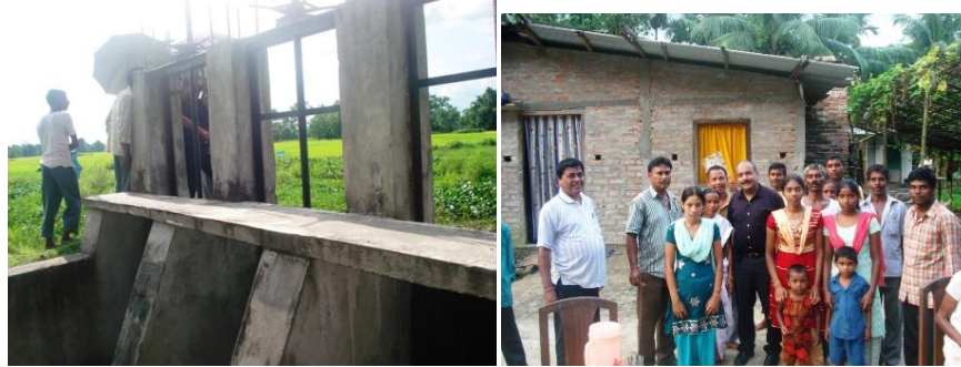
Christian Basti Flow irrigation project (Local Name: Kritupal Bheta ), Chirstian Basti, Sonitpur (Right: Happy faces of a minority farm family at the backdrop of their newly constructed pucca home”
